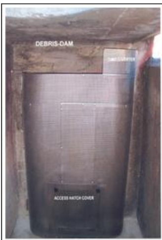
American Stormwater Debris Dam
